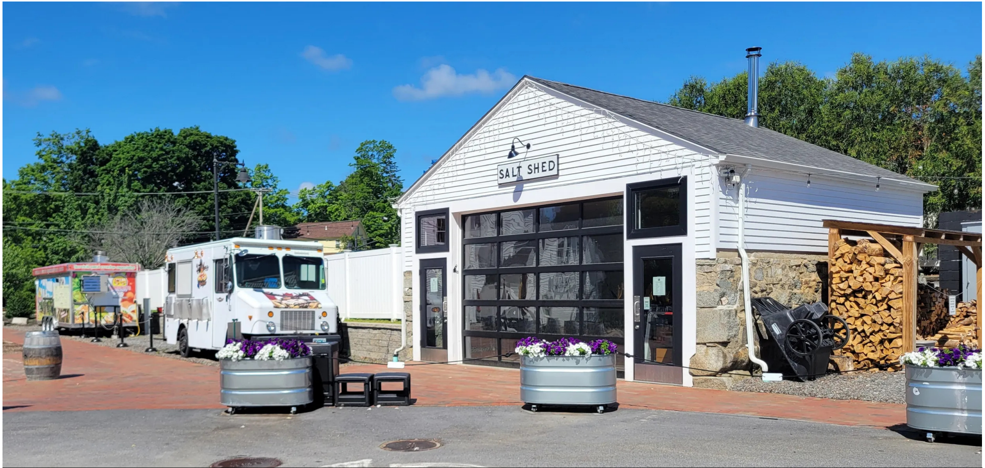
BUILDING 2 Salt Shed - 576 SF
